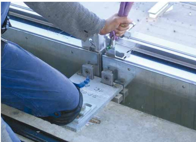
Glass façade to bracket connection
