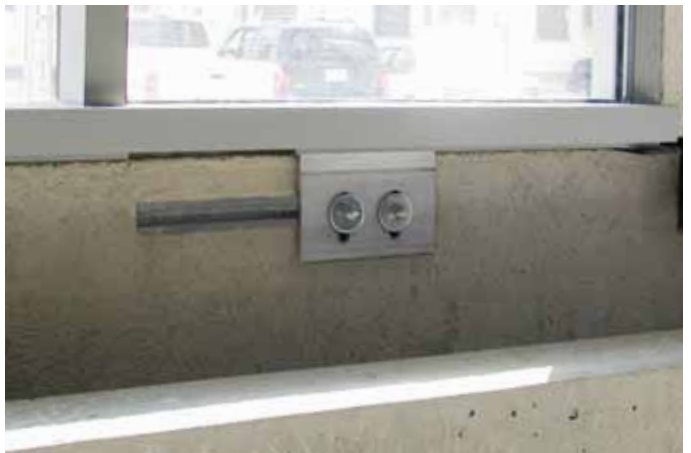
Window to sill-panel connection using a HALFEN Anchor Channel
