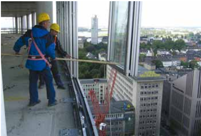
Installation of glass façade elements
