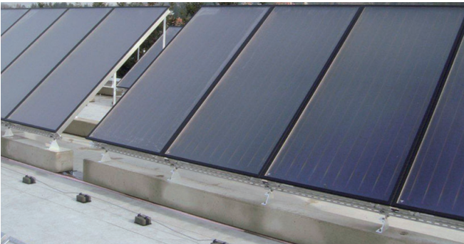
FIXING OF SOLAR PANELS
