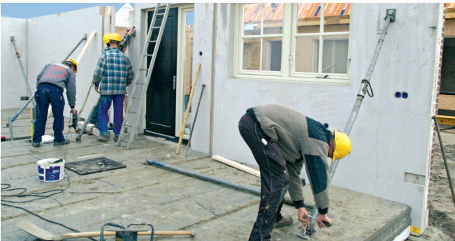
FIXING OF PROPS ON PRECAST ELEMENTS
