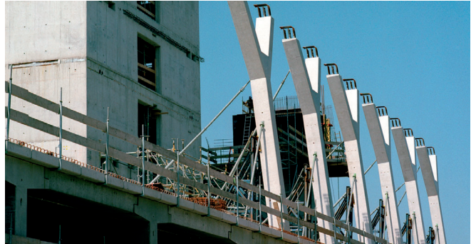
FIXING AND ADJUSTING PRECAST ELEMENTS
