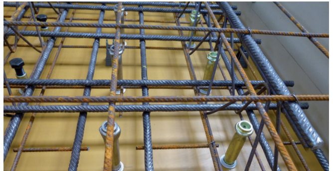
INSTALLATION OF FIXING ANCHORS
