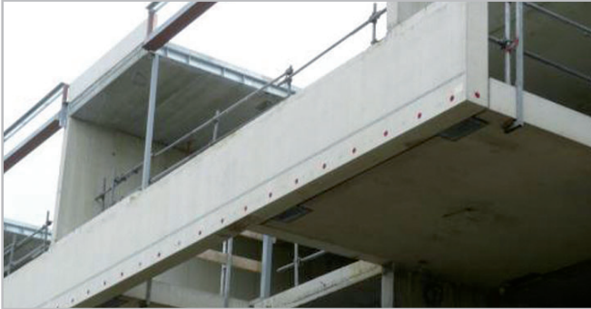
FIXING OF BALCONY RAILINGS
