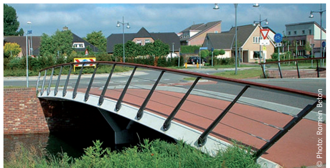
FIXING OF BRIDGE RAILINGS
