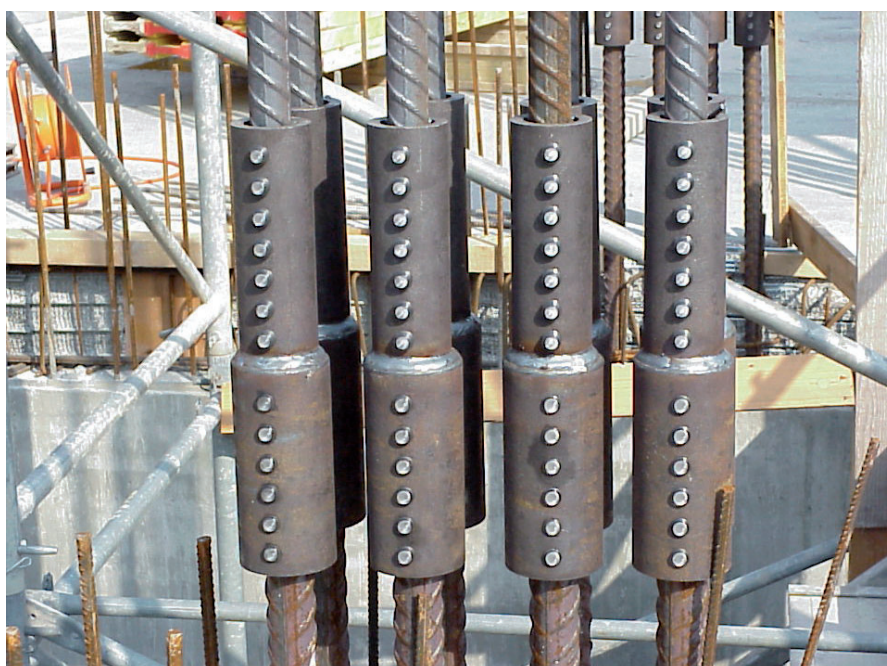
Support column with transition couplers
