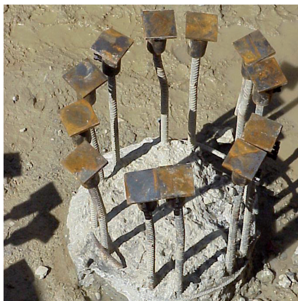
End zone detail in one pile
